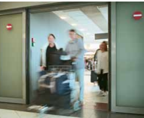
Automatic fire protection door, baggage claim, LYS
