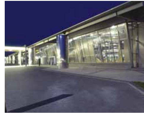
Automatic doors, facade, BLL
